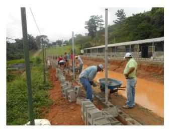
The hatchery construction team laid block around the perimeter of the new hatchery.
